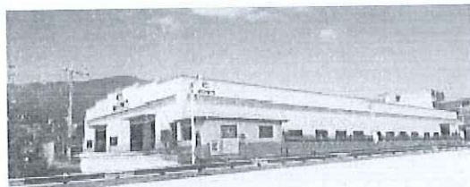
◎ 铁附件生产车间 Iron accessories production workshop
