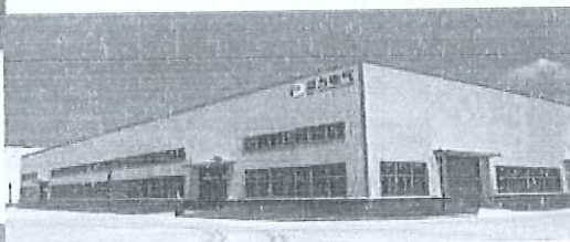
◎ 铁塔生产车间 Tower production workshop
