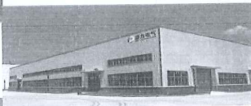
● 铁塔生产车间 Tower production workshop
