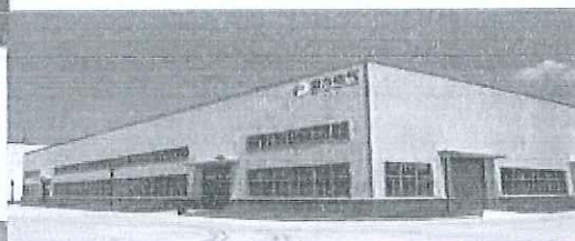
● 铁塔生产车间 Tower production workshop
